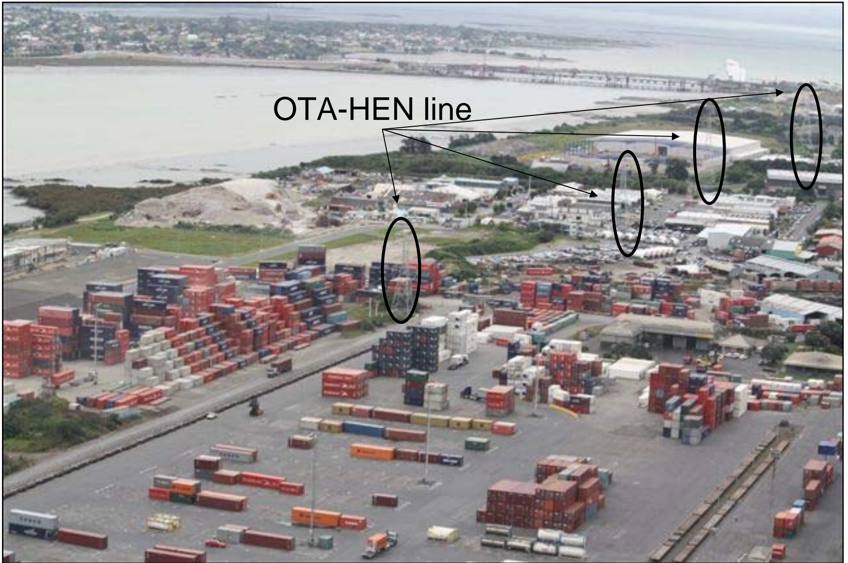
Metrobox container storage yard, Onehunga
