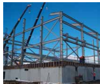
New gas insulated switchgear (GIS) facility under construction at Otahuhu.
